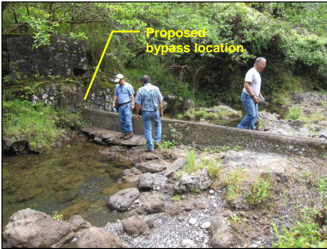
Diversion dam facing the left bank of West Wailuaiki Stream.
