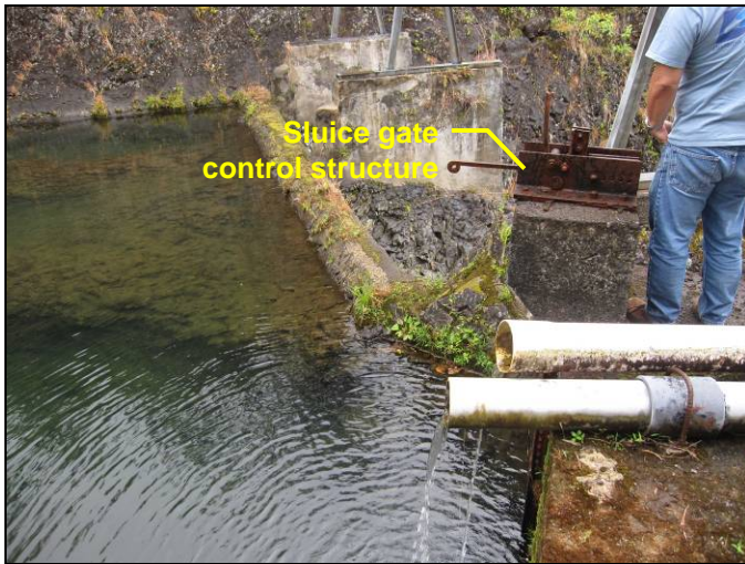
Diversion dam with minor diversion pipes in the foreground.
