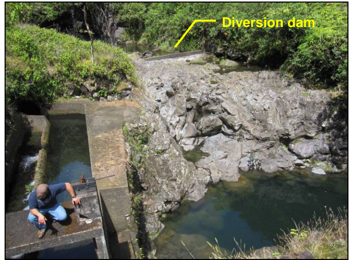
Upstream view of sluice gate/intake structure (left) and dam (center).
