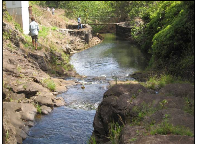
Downstream view from above the New Hamakua Ditch intake bypass.
