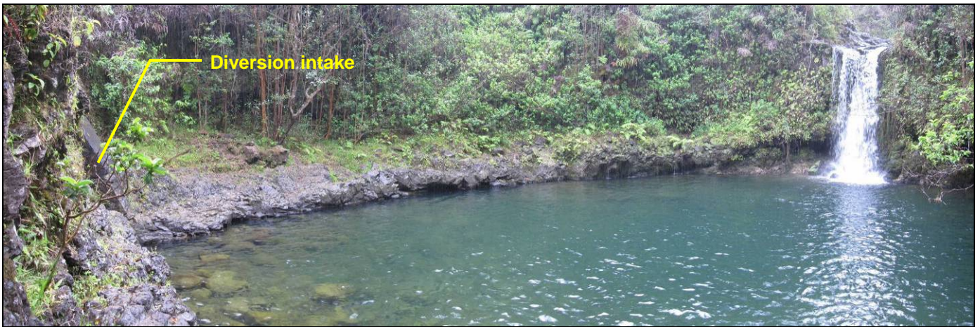
Panoramic view of right bank of Waiohue Stream with waterfall and diversion intake (left), and possible location for bypass pipe installation.
