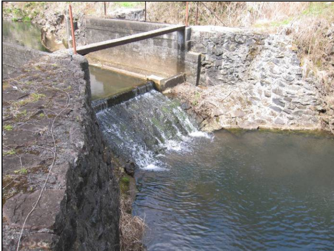
Overflow bypass from the New Hamakua Ditch diversion intake.
