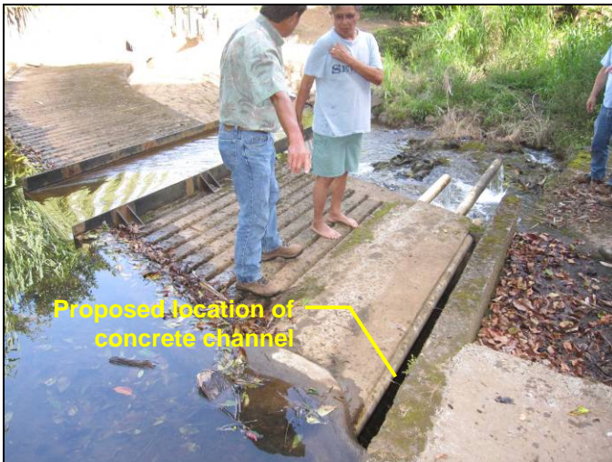
Right bank of the Haiku Ditch diversion intake on Honopou Stream.
