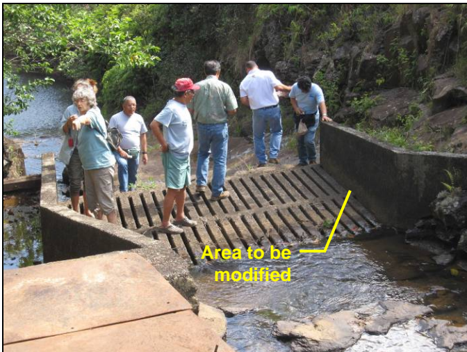
Downstream view of the Wailoa Ditch diversion intake.
