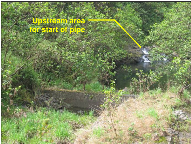
Diversion dam on the right bank of East Wailuaiki Stream.
