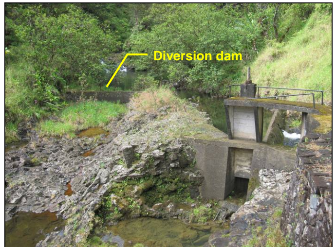
Upstream view of dam (left) and sluice gate/intake structure (right).
