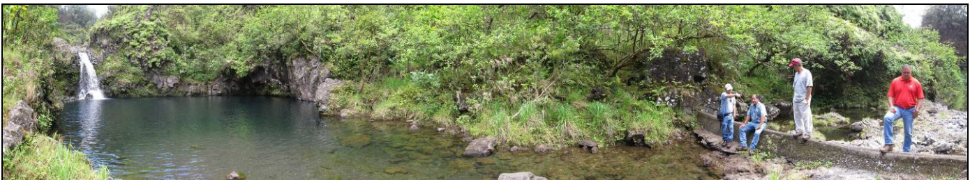
Panoramic view of left bank of West Wailuaiki Stream with waterfall and diversion dam (right), and possible location for bypass pipe installation.
