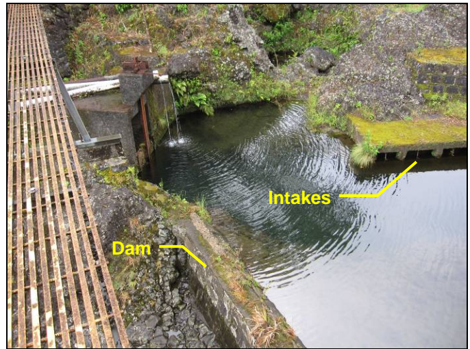
View from the opposite (left) bank of Hanawi Stream.
