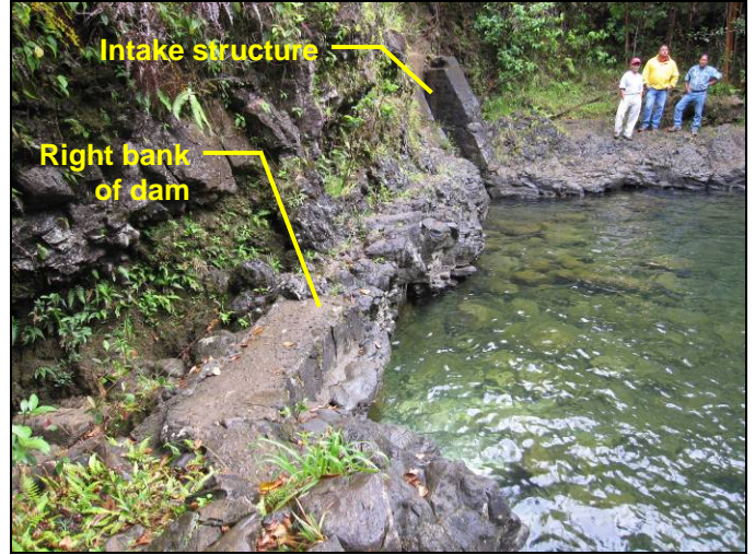
Diversion intake and dam structure on Waiohue Stream.
