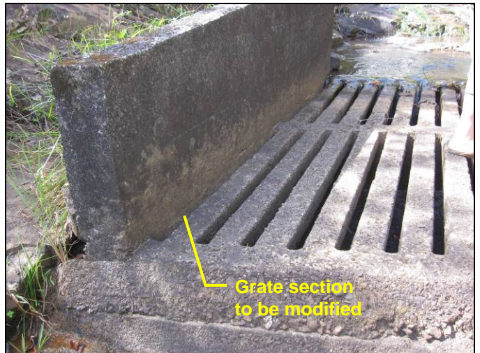
Close-up of the right bank of the Wailoa Ditch intake grate.
